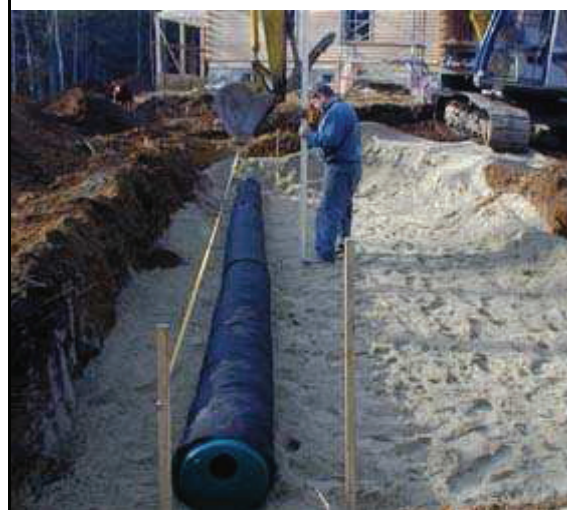
Enviro-Septic® being installed following the hydraulic linear loading rate
